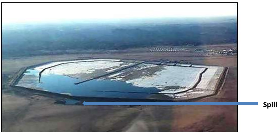
Figure 51: Husab Mine Tailings Facility with Water Spill
