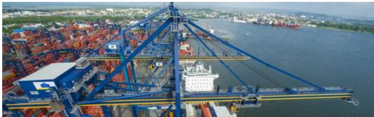
Figure 14: Ship-to-Shore Cranes as Purchased by Namport
